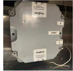
Note: There is a disconnect toggle on the right side of the junction box. The unit will be shipped to you with the toggle in the OFF position. Once you have hooked up the electrical source ensure you flip the toggle to the ON position to electrify the unit.
