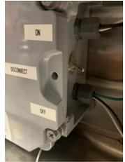
This electrical source can be brought in from the bottom (base) of the freestanding unit. Alternatively, holes can be drilled into the structure to allow the electrical to come through the side or rear of the freestanding unit.
